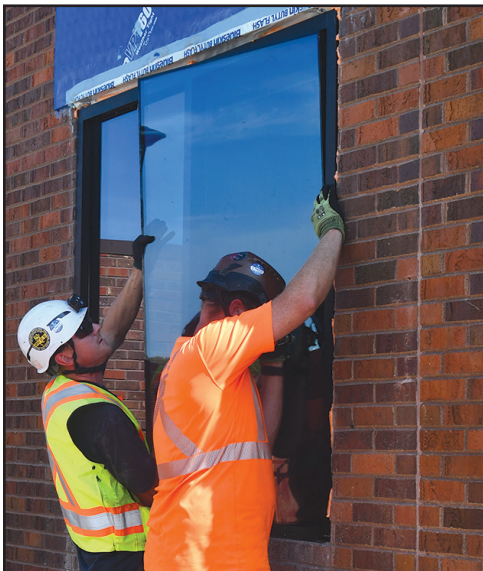
Window installation started August 17.
