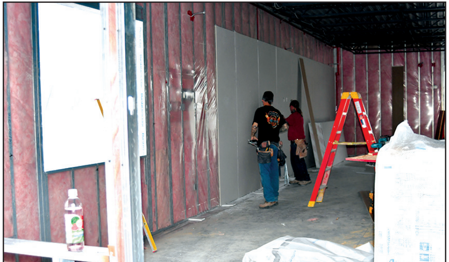
Insulation, vapor barrier, sheetrock and taping occurred in the new employee lunchroom/meeting room August 14.
